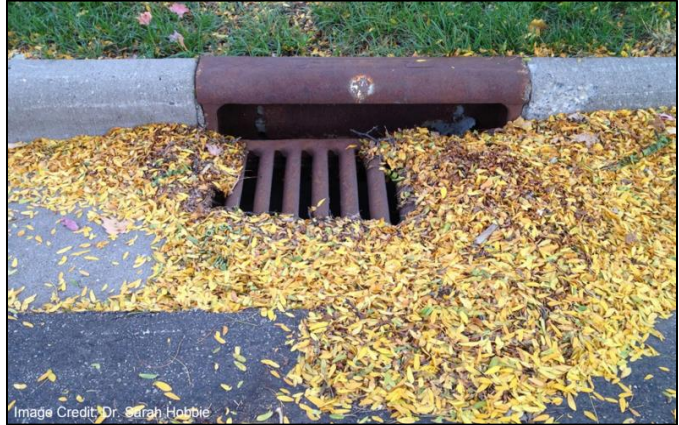
Figure 1. Leaves, seeds, and other tree debris accumulating in road gutters will eventually wash into storm drains and downstream waterbodies unless they are removed.
