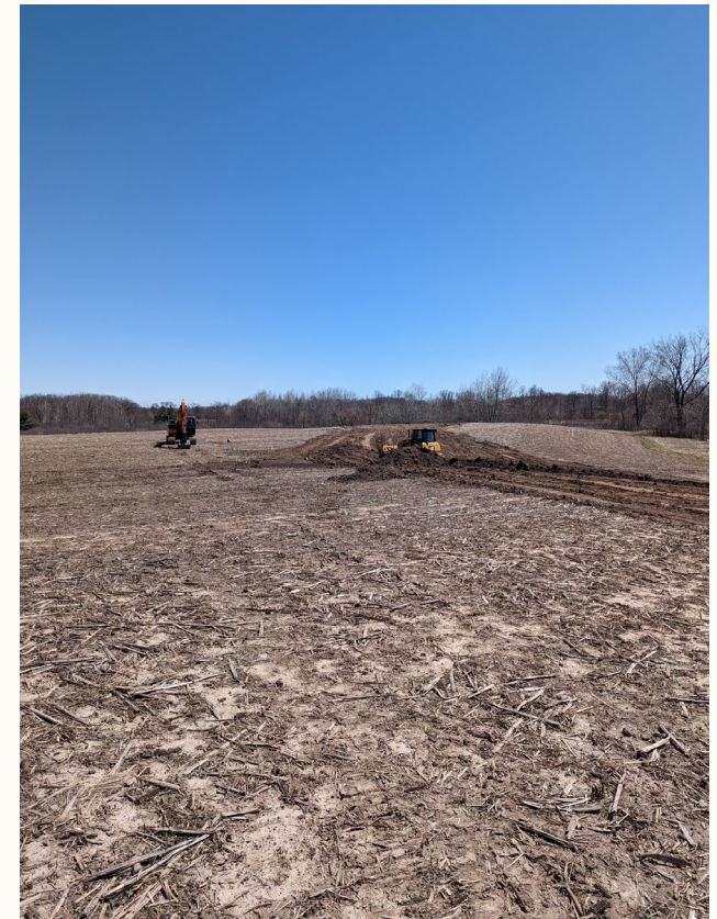
Construction of WASCBs
